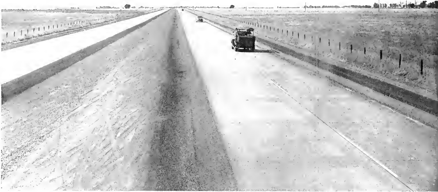
View of typical section of 4-lane divided highway on partially completed Davis-Dixon cut-off recently opened to traffic
